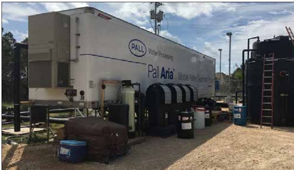
Figure 3. Temporary Trailer-Mounted Pall Water Aria FAST Membrane System Installation in New Braunfels, Texas
